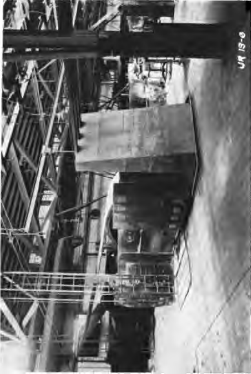
Various forms of guards for main belts are shown on this page.
